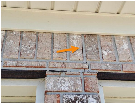
Garage at driveway
