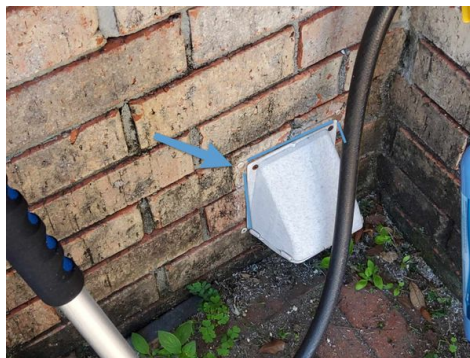
Caulk at vent
