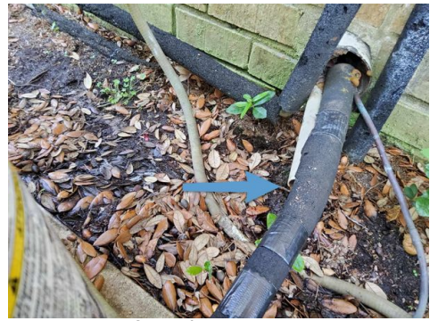
Drain away from house
