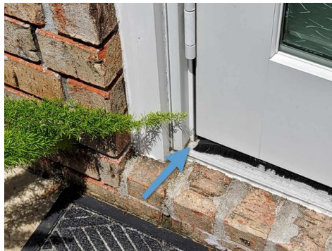
Rear bath exterior door
