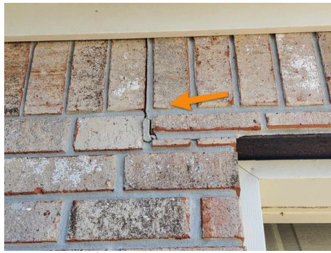
Garage at driveway
