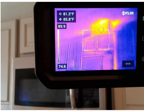
Exhaust fan chase at kitchen
